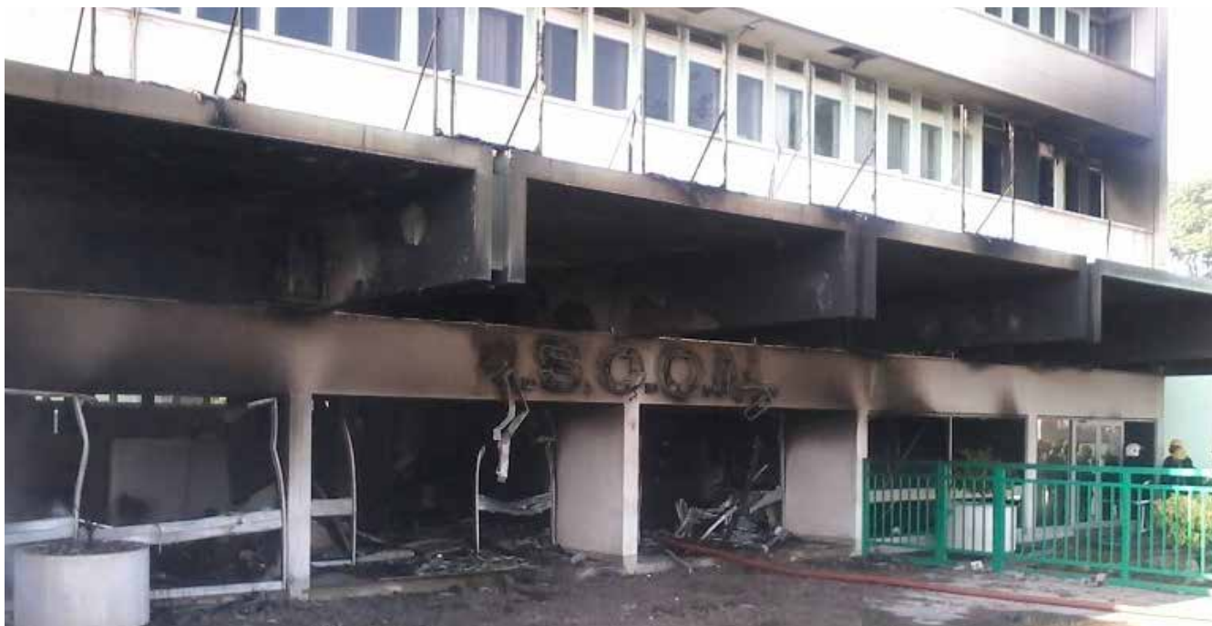
The ESCOM building whose demolition contract was cancelled
