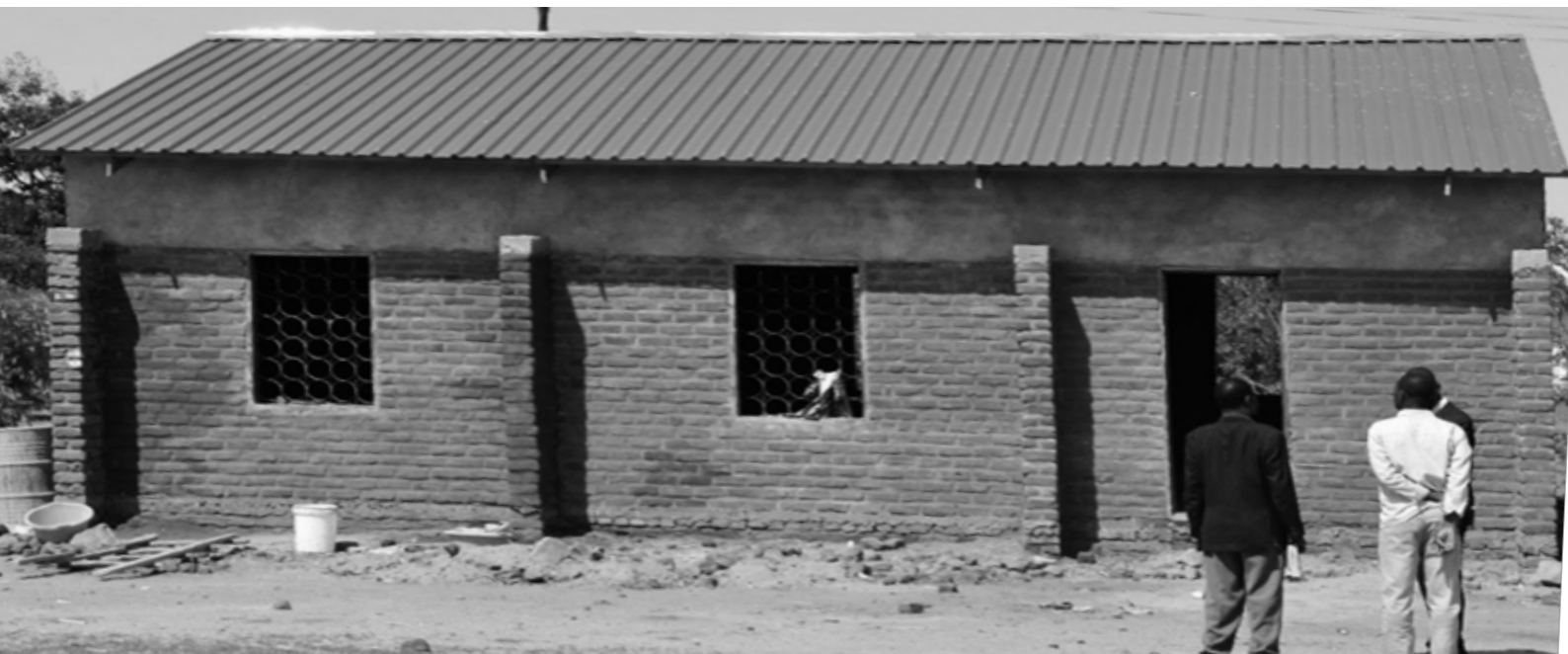
CHRR Community monitors at the completed classroom block at Linthipe Primary School.
